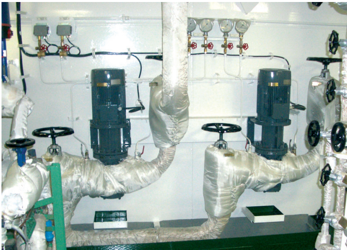
Abb. 2 Fuel Oil Feeder and Booster Pump L3NG with Magnetic Coupling
