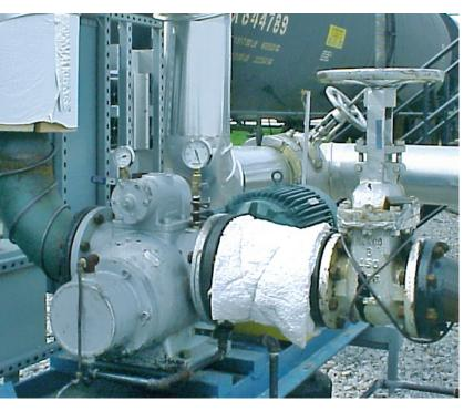
Installation of L2 pumps for railcar unloading
