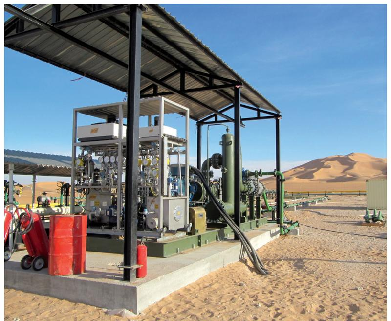
Fig. 2: Multiphase pump in Algeria
